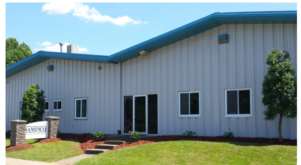
Our Huntington, WV facility includes our panel shop, rebuild / repair workshop, and motor warehouse.
